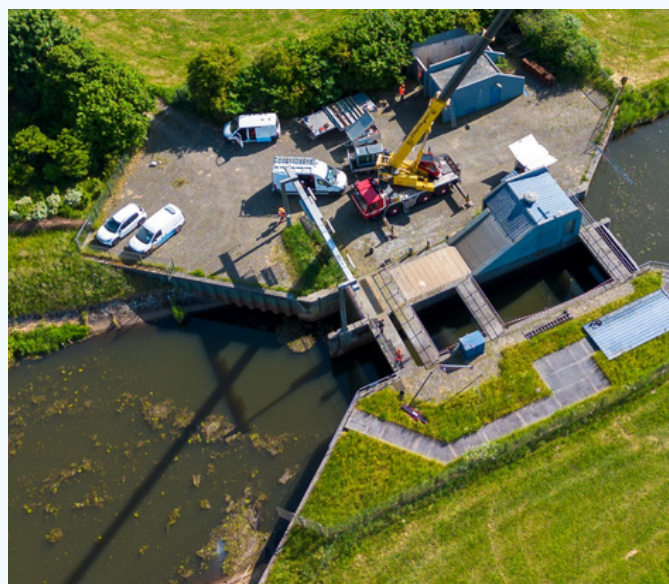
Rietberg pumping station Source: WDODelta
